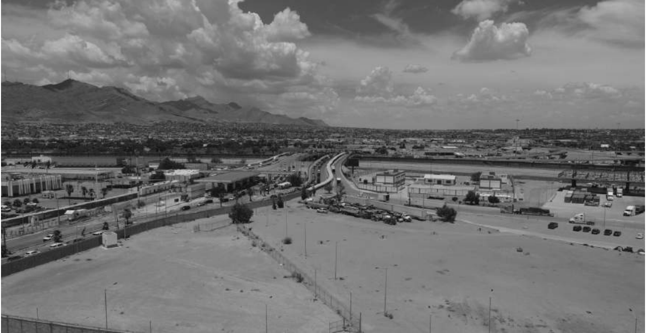
Bridge of the Americas PoE located in El Paso, Texas
