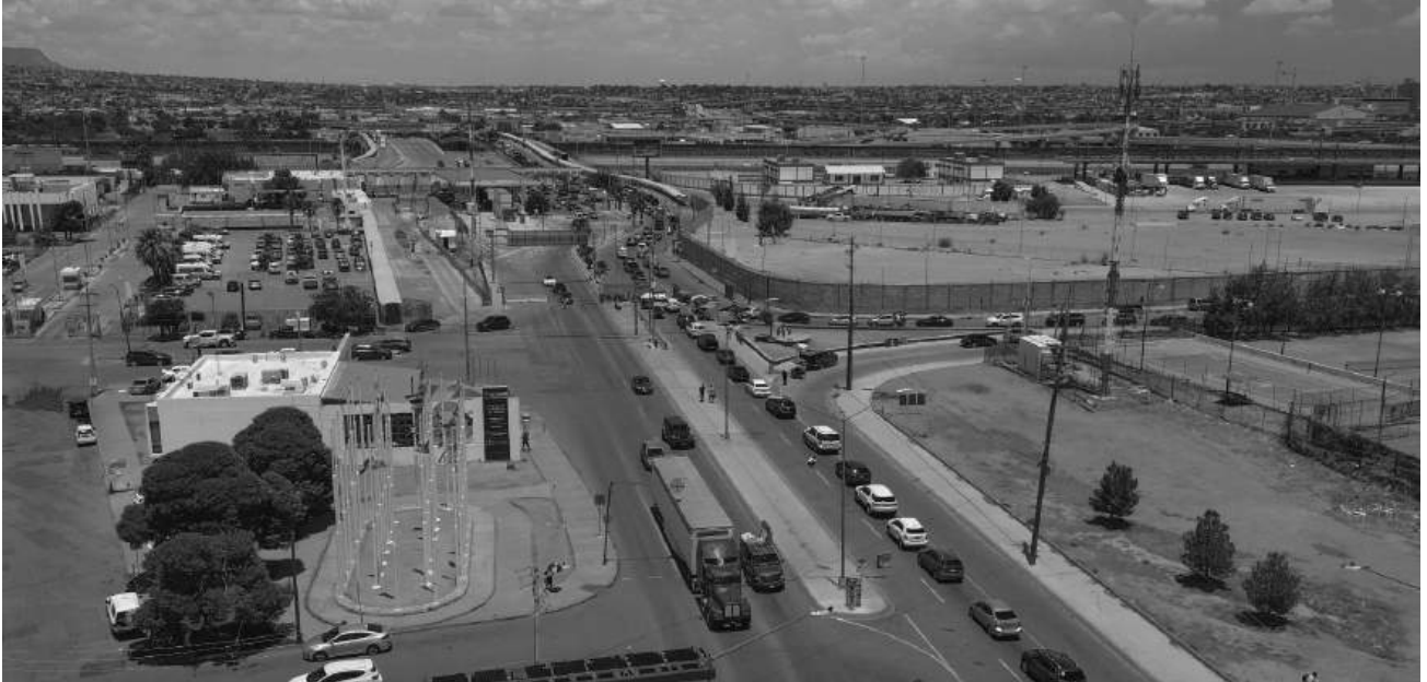
Bridge of the Americas PoE located in El Paso, Texas
