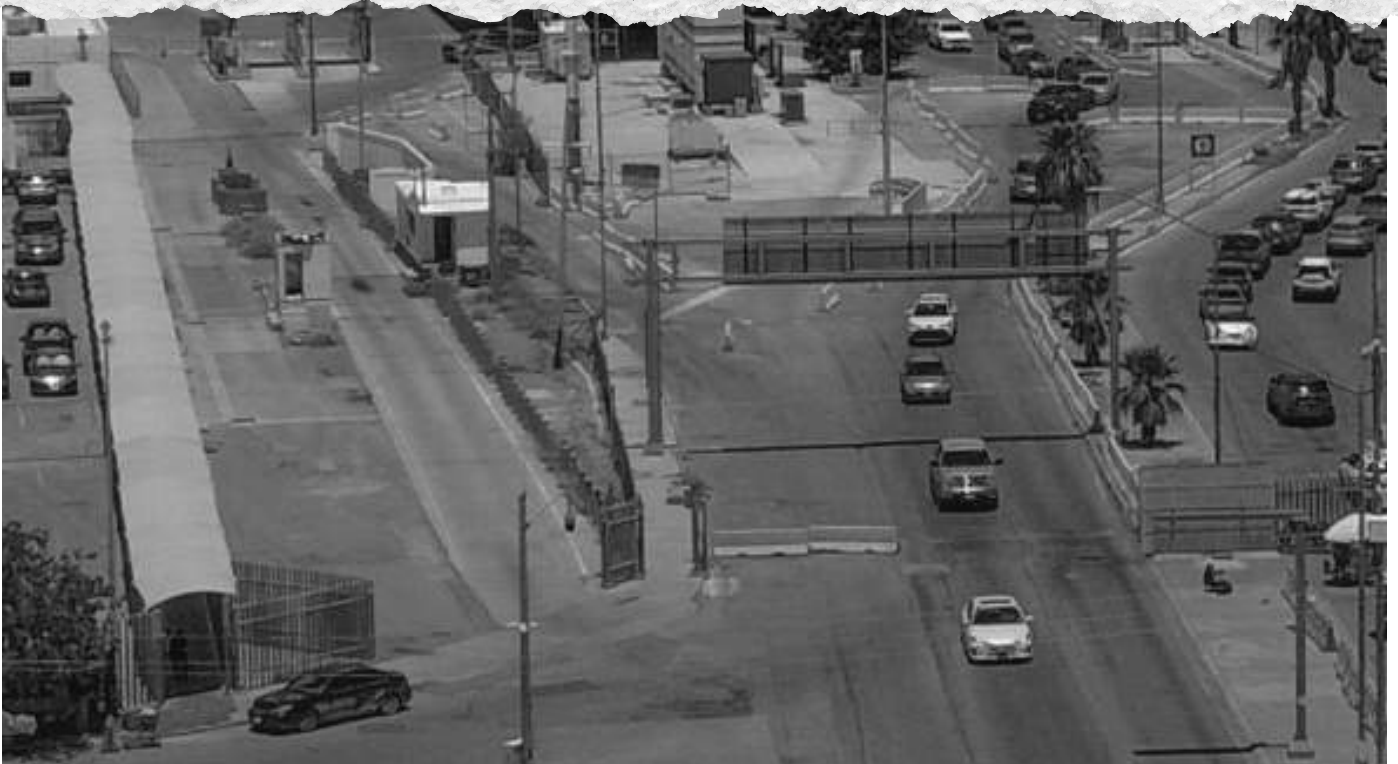
Bridge of the Americas PoE located in El Paso, Texas
