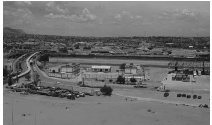
Bridge of the Americas PoE located in El Paso, Texas
