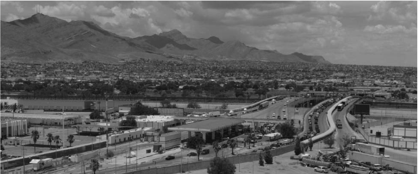
Bridge of the Americas PoE located in El Paso, Texas
